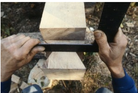
Wendell (Mass.) Bicentennial Celebration: cutting tenons for post and beam building 1981 wen157.jpg
