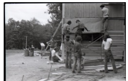
Group putting up clapboards on commune building (Warwick, Mass.)
