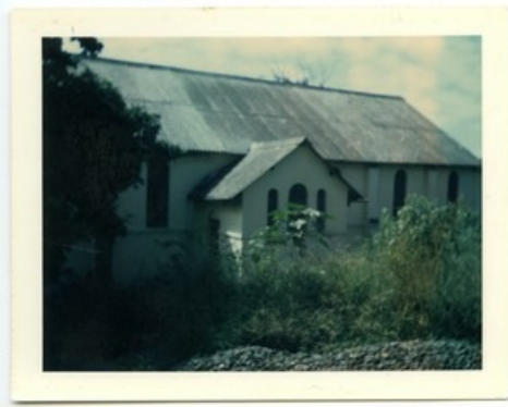
Groutville, cemetery behind the church
